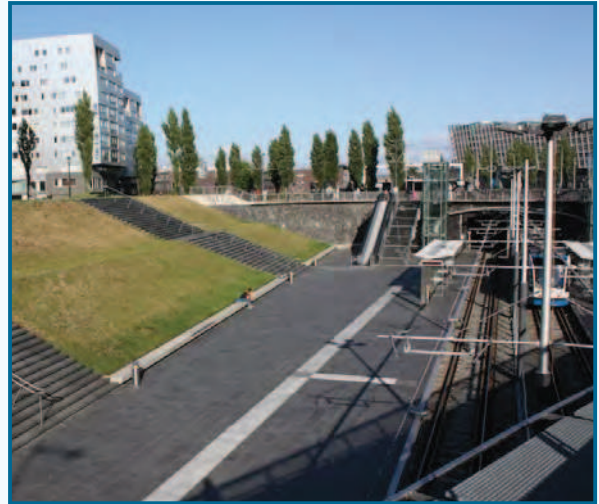
The new Reitlandpark railway station in a new district of Amsterdam demonstrates how a station separated by a change of level can be integrated into its surrounding urban context.
